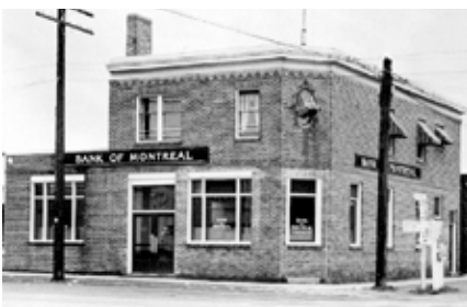
The Bank of Montreal building at a later time. Note the extension to the left.
