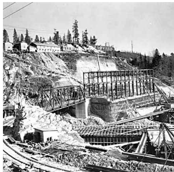
Powerhouse construction in April 1930
