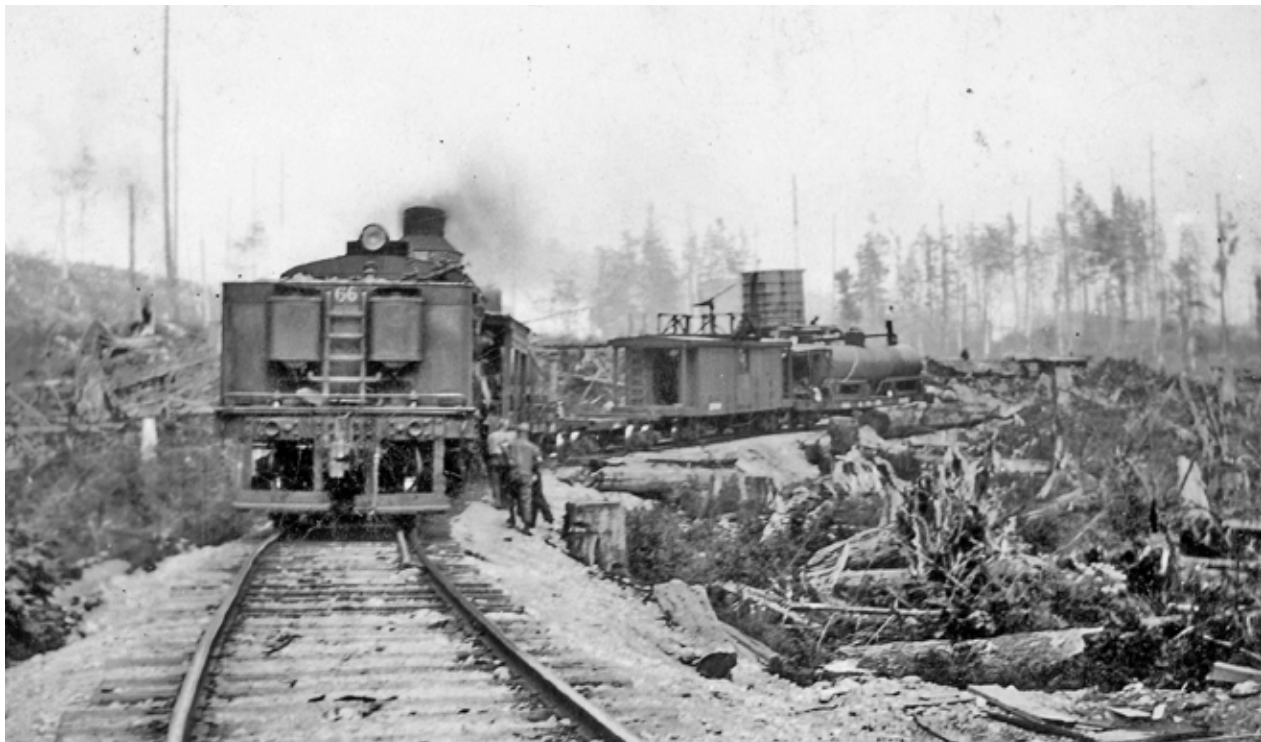
Abernethy & Lougheed main line to Gold Creek in about 1930. Train consisting of two locomotives (one is #66) and a couple of cars parked on track in middle of clear-cut. On back: "Taking on water to fight a fire... H.R.H. Edward Prince of Wales visited this camp in 1925.
